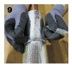
It is recommended to additionally secure the mineral wool pipe section with aluminium bands or soft galvanised binding wire.<sup>2)</sup>
