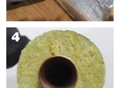
To minimize heat loss when installing horizontally, align the longitudinal seam so that it is at the bottom of the pipel <sup>1)</sup>
